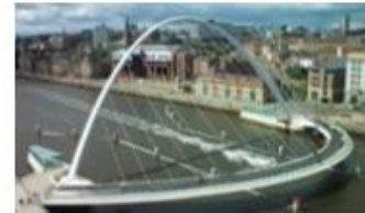
Millennium Bridge, Gateshead (Tilt)
