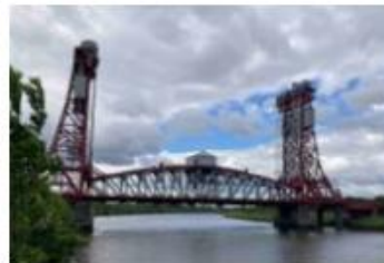
Tees Newport Bridge (lift)
